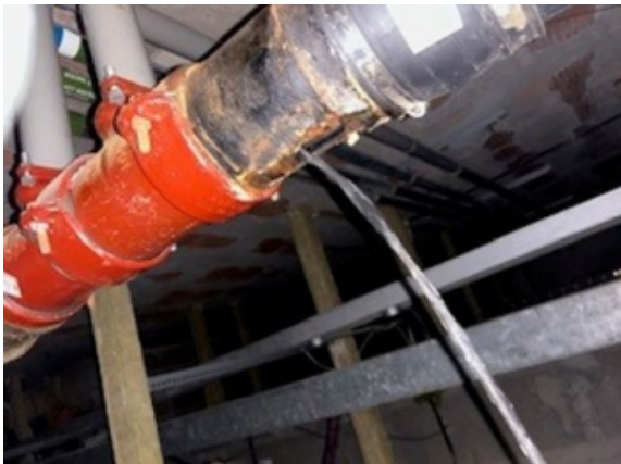
When the bathroom which the pipe was connected to was used, a strong stream of wastewater poured through the hole and into the roof space
