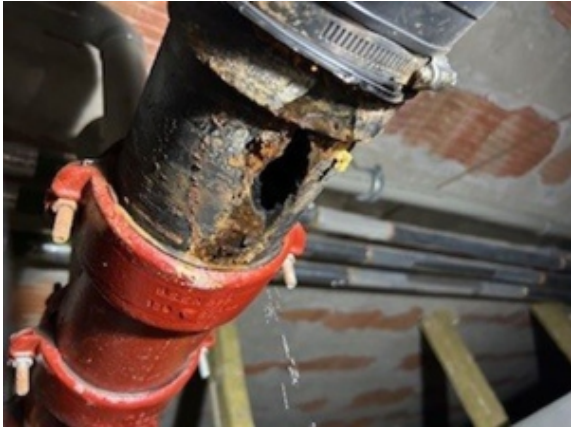
Corrosion caused an 80mm diameter hole to appear in the cast iron drain pipe which ran horizontally through a roof space in the hospital
