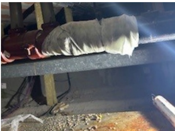
SylWrap HD was applied covering a 300mm section of the pipe, either side of the hole which was sealed using Superfast Steel Epoxy Putty
