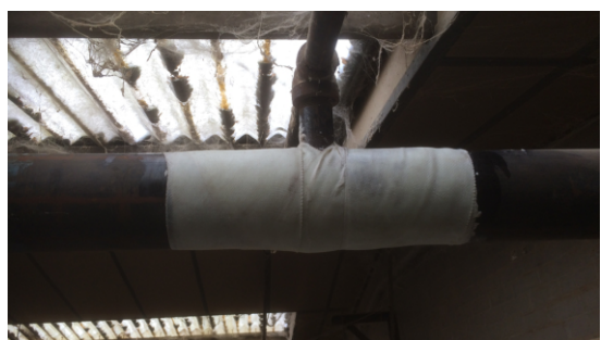
The completed repair carried out using Superfast Steel Epoxy and SylWrap HD Pipe Repair Bandage
