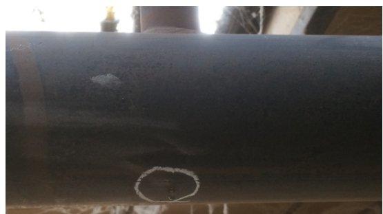
The pinhole leak was located underneath a tee, ruling out a repair using a clamp
